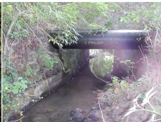
Figure 3 aval de la station
