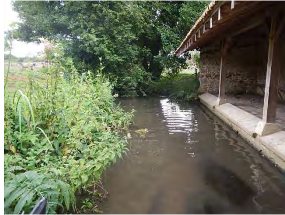
Figure 3 : aval de la station
